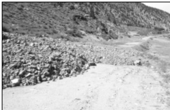
Smaller debris flows frequently cause loss of service on Colorado roads. Two examples this past summer were multiple events on I-70 near Dotsero and several debris flows on the frontage road west of Interstate 70 at Georgetown (shown above). PHOTO BY JIM SOULE
