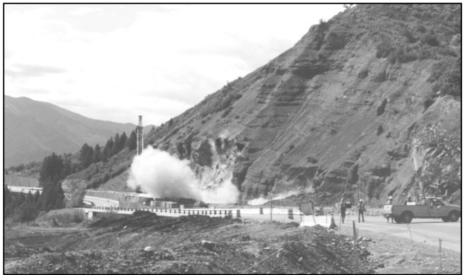
Blasting Highway 82 re-alignment at Shale Bluffs PHOTO BY R. PIHL
