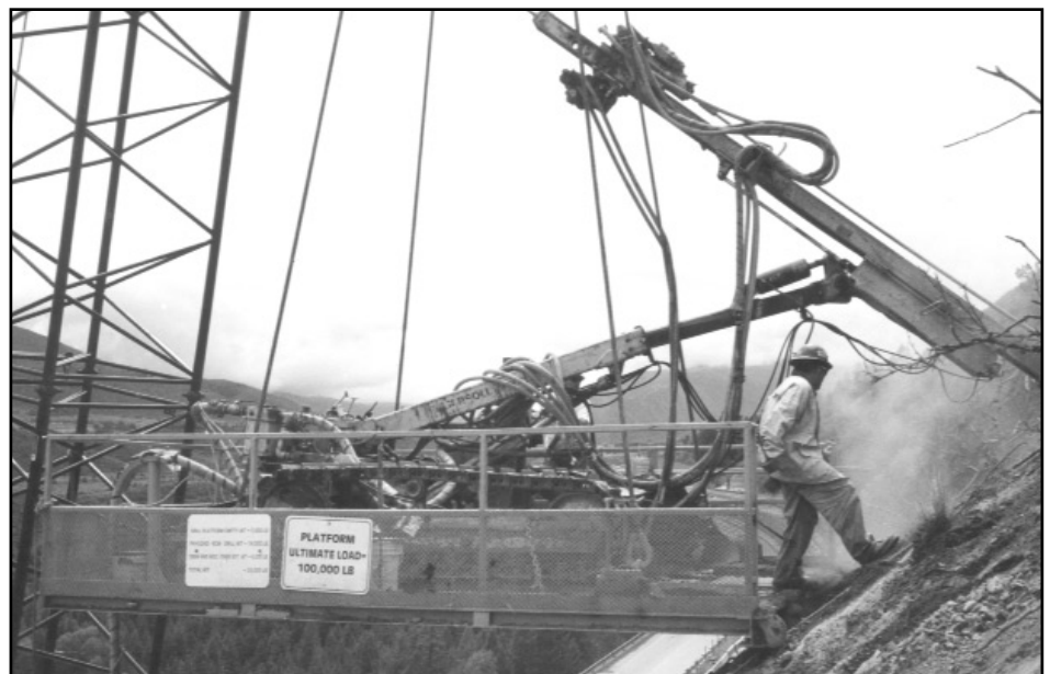
Rock anchor installation to support Mancos shale at CDOT Highway 82 Shale Bluffs project PHOTO BY R. PIHL
